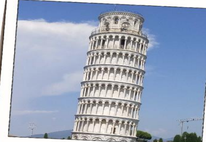
Leaning Tower of Pisa
